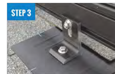
ATTACH L-FOOT TO RAIL
